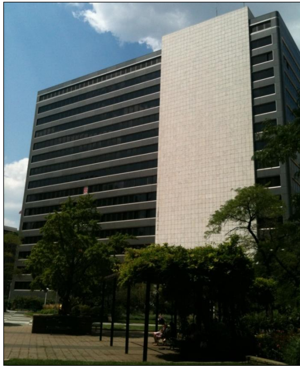
Figure 1 - Exterior Photo of River Vue Apartments
